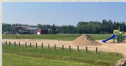
Improvements being made to Memorial Park in July
